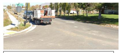
Segment is newly constructed. Access is adequate on South end. The asphalt widths are within the City Code standards except for the last 180 feet on the North end.
