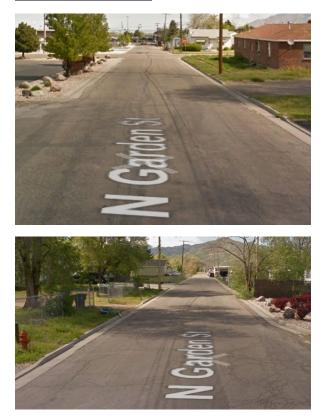
This section has curb and gutter throughout with about 26 feet of asphalt for the entire segment. With the gutter pan included the hard surface increases to 30 feet. There are 3 hydrants along this segment that are within code distances.
