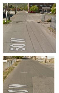
This section has been improved for the most part as well. Asphalt widths are at about 26 feet throughout this section.
